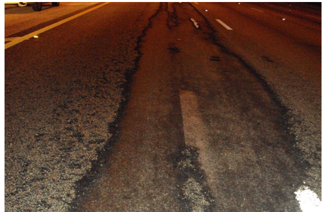
Figure 5: Example of ravelling
